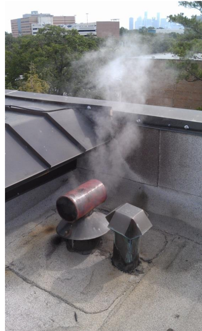
Sample project: Leaky pressure relief valve on roof repaired, preventing loss of steam
