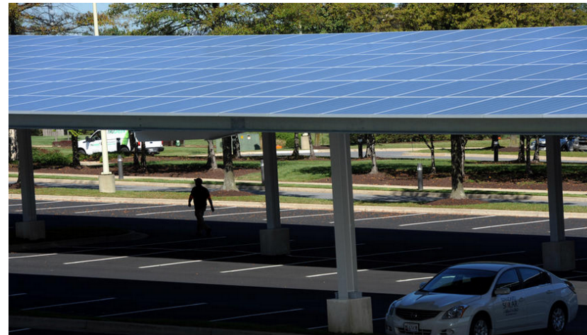
3. Carport-Mounted Solar Panels
